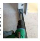
Fix the NO-AIR floor plugs with finned gasket on both sides with the screws from the brace.
