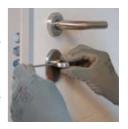
Remove the plate around the cylinder with the aid of a screwdriver
